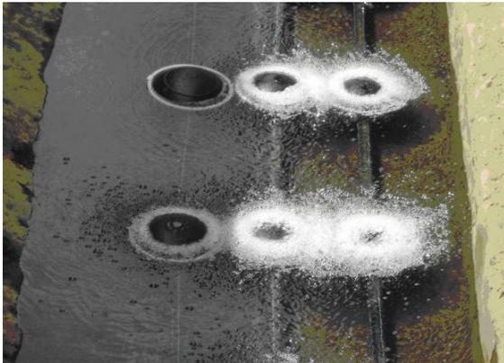
Fig. 6.1, The operating of porous diffusers at a minimum level of water in the basin.
