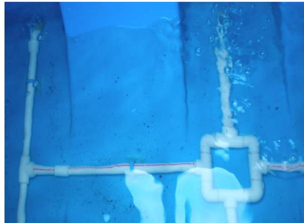
Aeration system using perforated pipes
